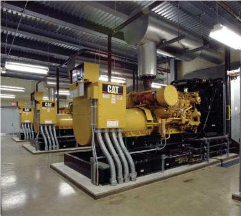
Cat generators standby in case an outage exceeds the capacity of the flywheel UPS system.
