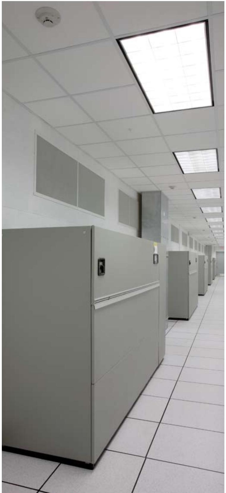
*Jackson still wanted to maintain a finished look via a lay-in ceiling, even though data rooms where cabling is routed overhead typically don't have ceilings.*
